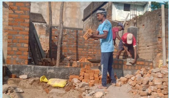
PMI House Construction for Jeeta Beuro, Odisha
