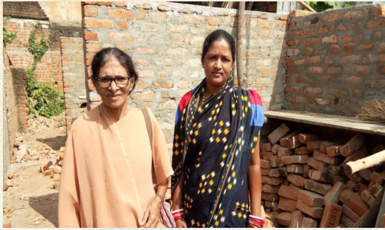
PMI Housing Project in Odisha in Progress
